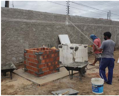
Figure 1: Prototypes under construction
