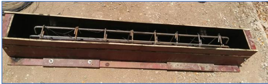
Fig. 3: Laying Reinforcement into wooden mould
