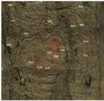
Figure 9: Concrete flow in highly dense reinforcement areas [7]
