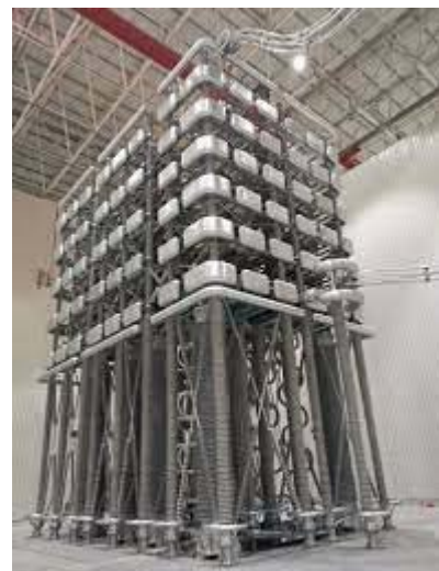
Figure 5: 500 kV hybrid HVDC circuit breaker
