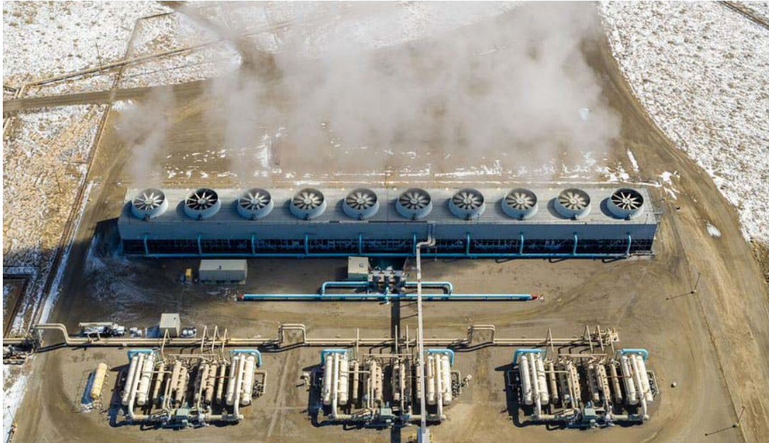
Fig. 4.5.1: Fervo Energy's 3.5-megawatt enhanced geothermal plant in Nevada. Credits to Google/Fervo Energy
