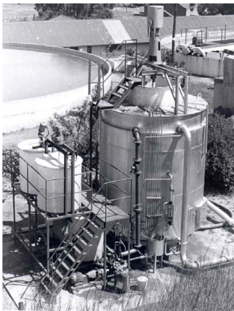
Figure 21: Installation of the second pilot HR clarifier at the municipal waterworks of the City of Bethlehem
