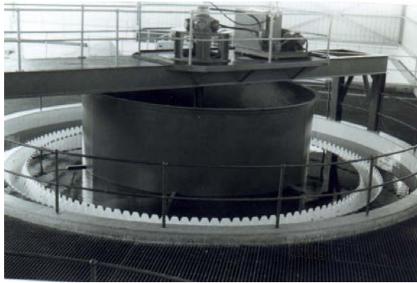
Figure 23: The Saulspoort waterworks – the HR clarifier, design capacity 10 \text{ ML.d}^{-1}
