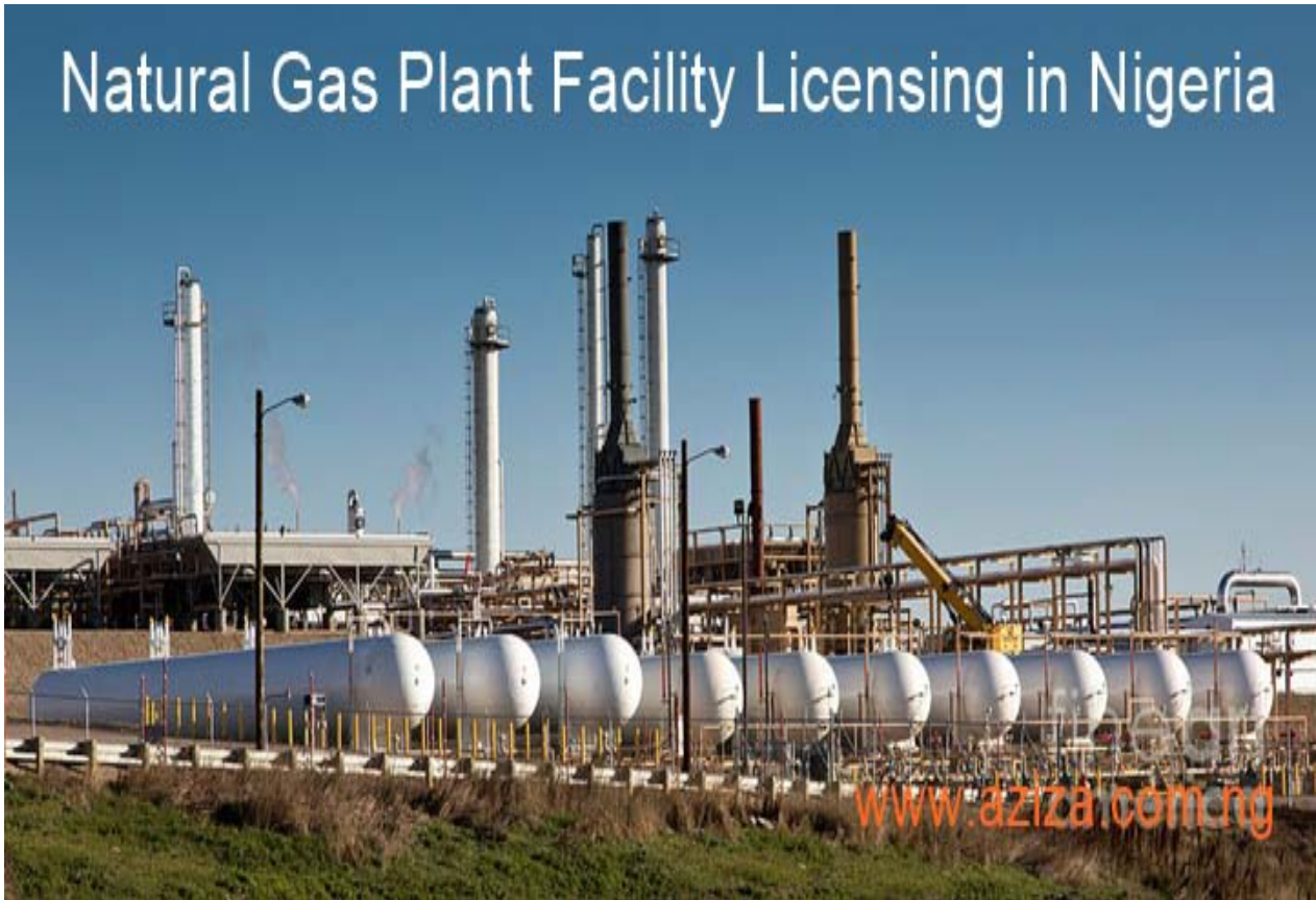
Fig. 1: Natural gas plant
