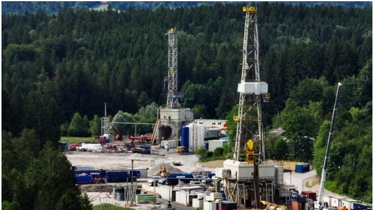
Fig. 4.5.3: Eavor Technologies Secures Major Investment from Kajima for Geothermal Advancement [57]. Credits to Eavor Energy
