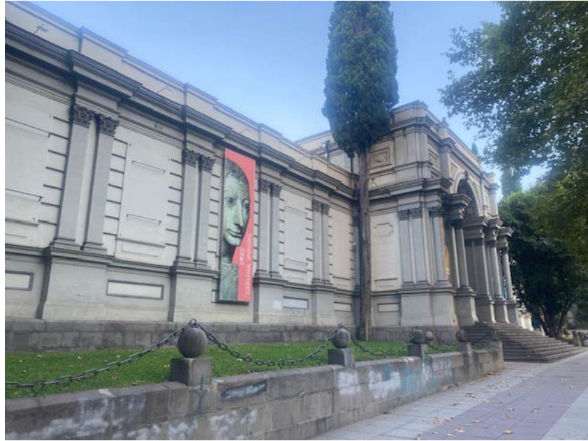
Fig. 14: National Gallery today from the side of Rustaveli Avenue
