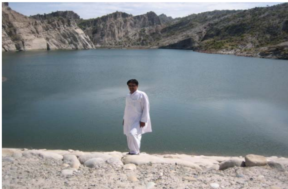
Fig. 7 : Small Dam for water storage at Sarki Lawager
