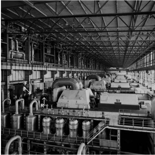
Fig. 1 : Machine hall interior with ten K-200 units (source: www.elturow.pgegiel.pl ). Letters F and R indicate front and rear HP turbine bearing of the foremost unit
