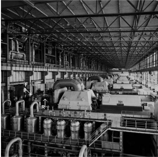
**Fig. 1 :** Machine hall interior with ten K-200 units (source: [www.elturow.pgegiel.pl](http://www.elturow.pgegiel.pl)). Letters F and R indicate front and rear HP turbine bearing of the foremost unit
