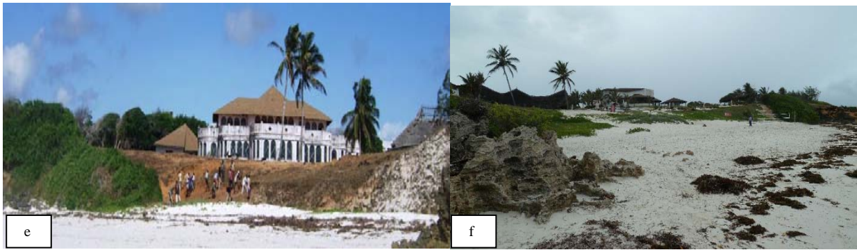
Figure 10: (a) Construction near HWM, (b) Impact of recreational activities along the beach, (c,d) construction of sea walls ,(e) (2007),(f) (2014)clearing of riparian vegetation and natural dune
