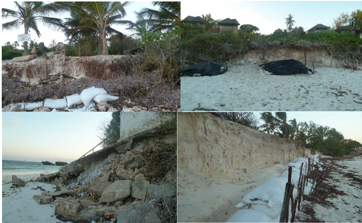
Figure 11 : Adjacent properties affected by erosion displaced by sea walls and other fortifications
