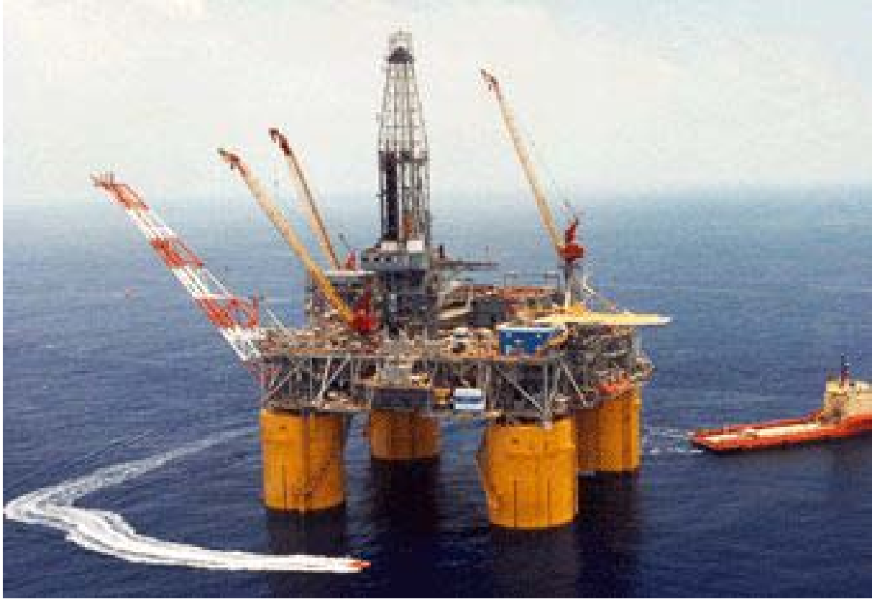
Fig. 3 : Mars Tension-leg platform in the Gulf of Mexico (From http://en.wikipedia.org/wiki/Mars_(oil_platform) )
