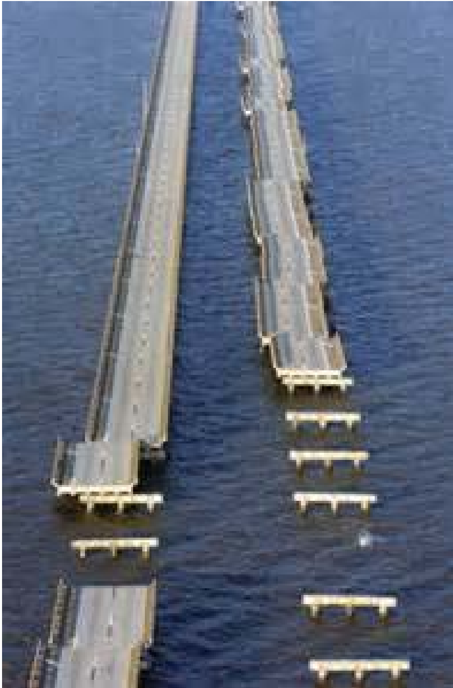
Fig. 5 : Interstate I-10 over Mobile Bay damaged by Hurricane Ivan in 2004(From FHWA-NHI-07-096).According to FHWA, the wave setup on top of the storm surge was the cause
