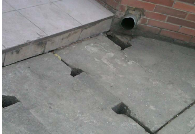
Plate 5 : Underground drains at Ibom Plaza
