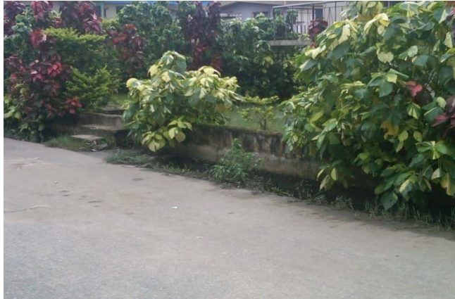
Plate 2 : Flood Control at Nsentip street flood area.z
