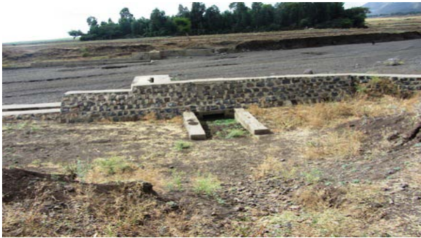
Intake structure of Hara scheme
