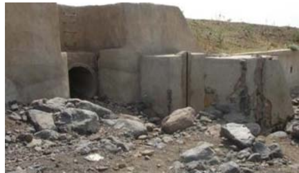
Orifice intake, Tirke scheme
