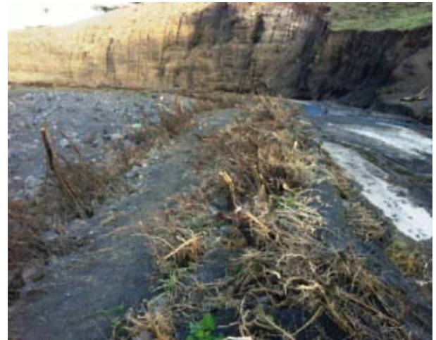
Embankment using forest and shrub, Oda
