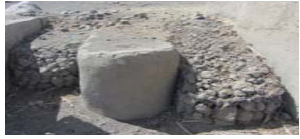
Sluice gate blocked by gabion, Tengago
