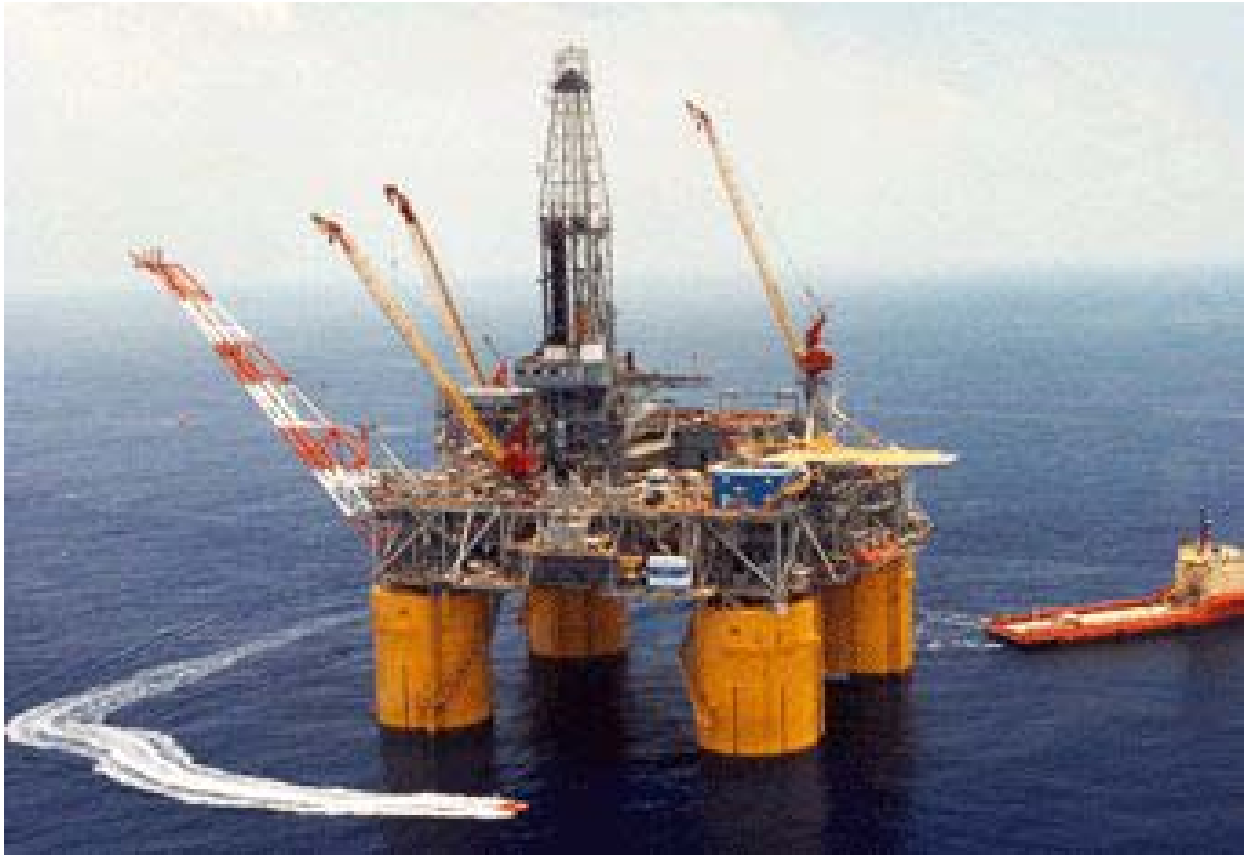
Fig. 3 : Mars Tension-leg platform in the Gulf of Mexico (From http://en.wikipedia.org/wiki/Mars_(oil_platform) )
