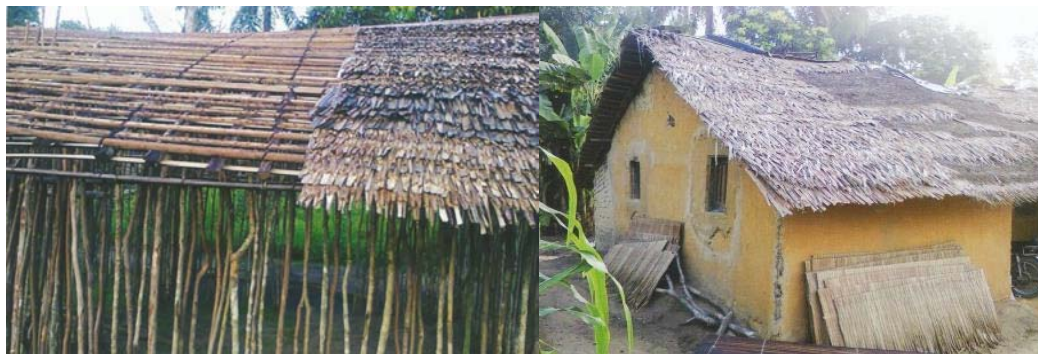
Figure 3 : Thatch Roof
