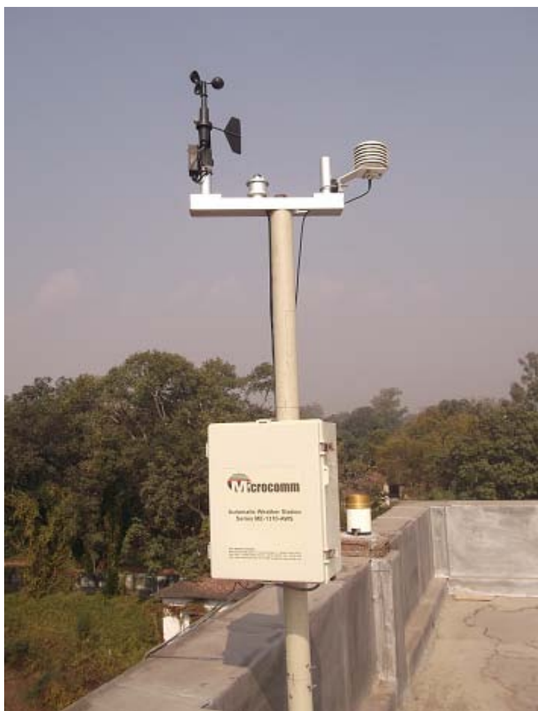
AWS (Automatic weather station)
