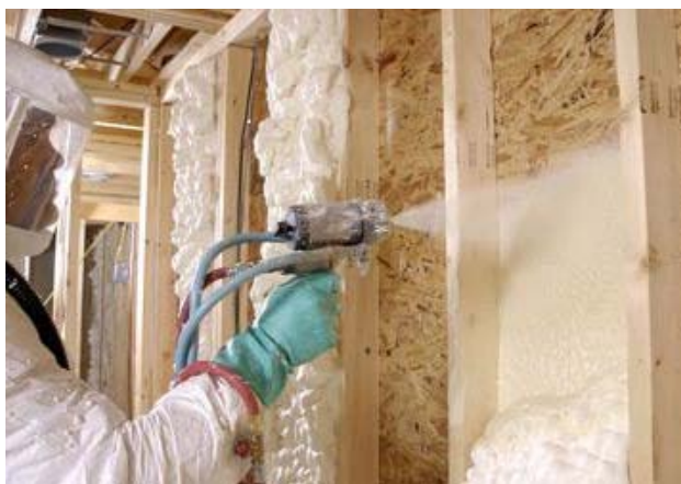
Figure 5: Application example of polyurethane foam
