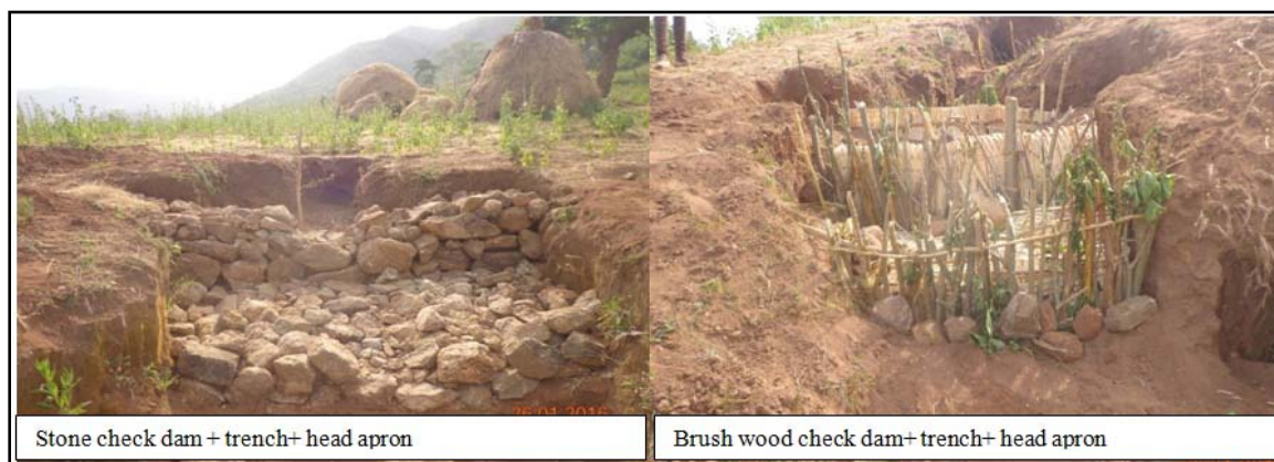
Figure 3: Gully treatments just after construction
