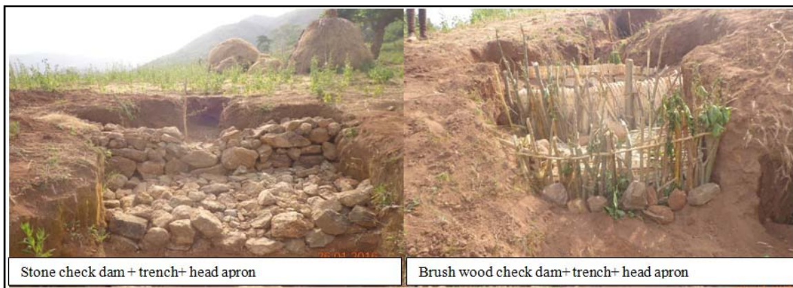
Figure 3: Gully treatments just after construction
