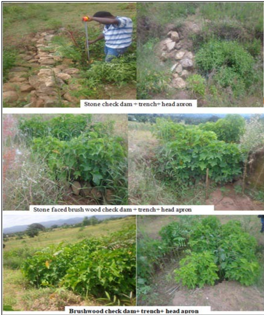
Figure 4: Progressive rehabilitation system of gully by different check-dams
