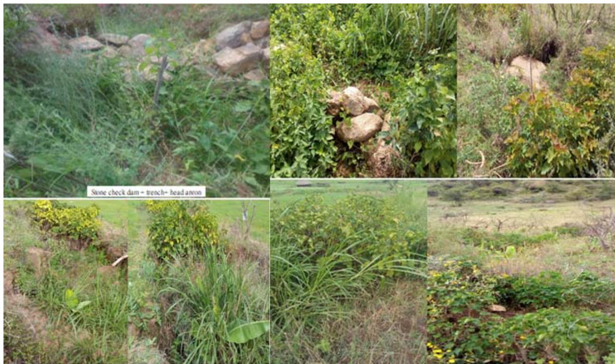
Figure 5: Gully stabilized with different check-dams and vegetative materials after two years
