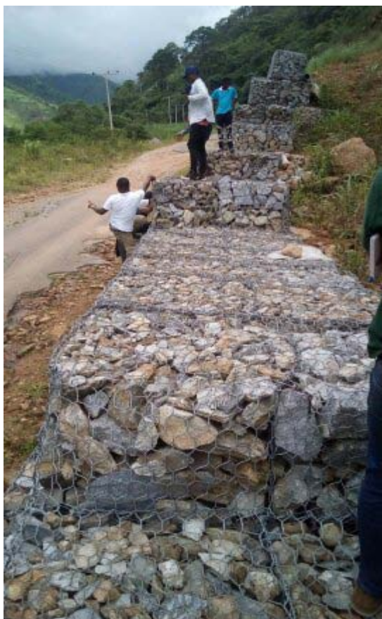
Plate 7: Rock netting a method for protecting critical infrastructure like road and human settlements near Obudu Plateau cattle ranch gate
