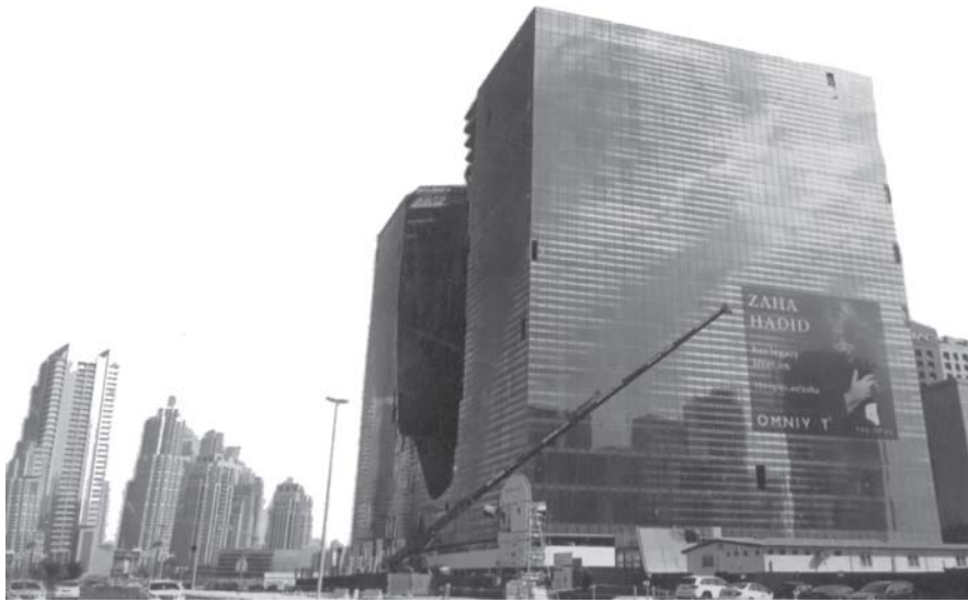
Fig. 15: The Opus Business Bay, Dubai (UAE), Architect Zaha Hadid. Materials used for facade and fenestration include aluminium unitized curtain wall system, steel and aluminium skylight system, carbon fibre composite stick system curtain wall and high-performance mirror fritted and blue body tinted double curved glass. The glazing comprises complex 3-D forms especially manufactured for the facade.
