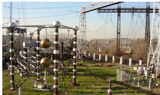
Figure 3: Test installation with a cascade of transformers for 1 million volts with a pilot span of an overhead line 500 kV 300 m long
