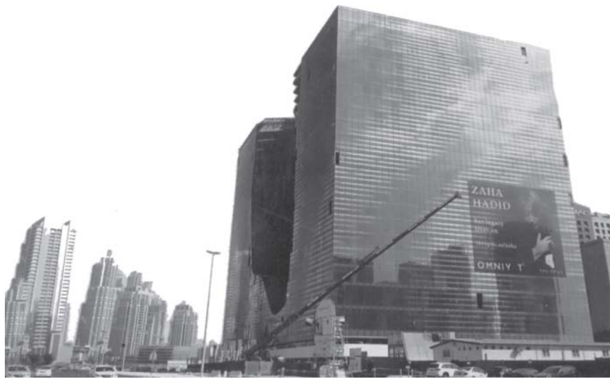
Fig. 15: The Opus Business Bay, Dubai (UAE), Architect Zaha Hadid. Materials used for facade and fenestration include aluminium unitized curtain wall system, steel and aluminium skylight system, carbon fibre composite stick system curtain wall and high-performance mirror fritted and blue body tinted double curved glass. The glazing comprises complex 3-D forms especially manufactured for the facade.
