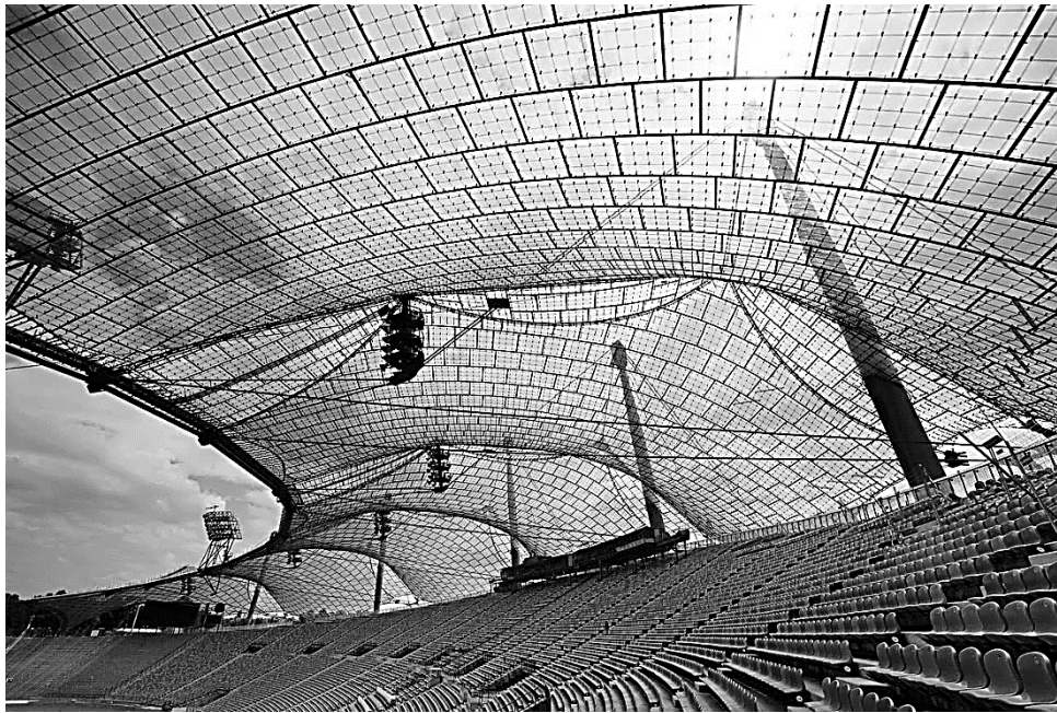
Fig. 22: Frei Paul Otto used lightweight tensile and membrane structures in the roof of the Olympic Stadium in Munich for the 1972 Summer Olympics
