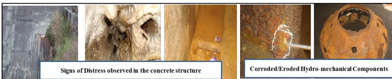
Figure 4: Signs of distress observed in the concrete structure and various other components
