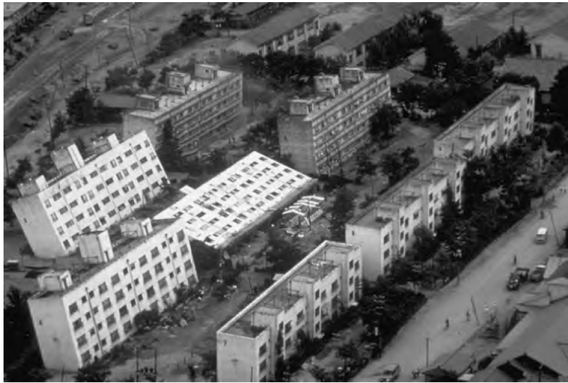
Figure 1: Tilting of Apartment Buildings Caused by the 1964 Niigata Earthquake.
